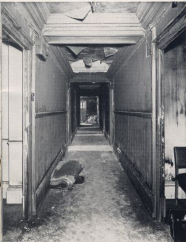
Sixth floor corridor.
