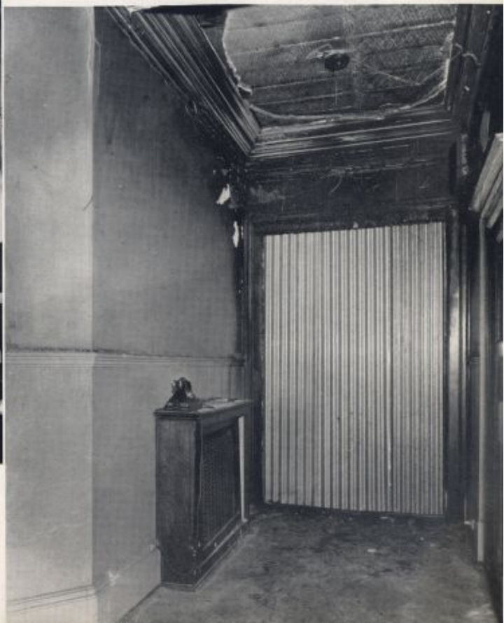
Third floor entrance sealed off from the main staircase.
