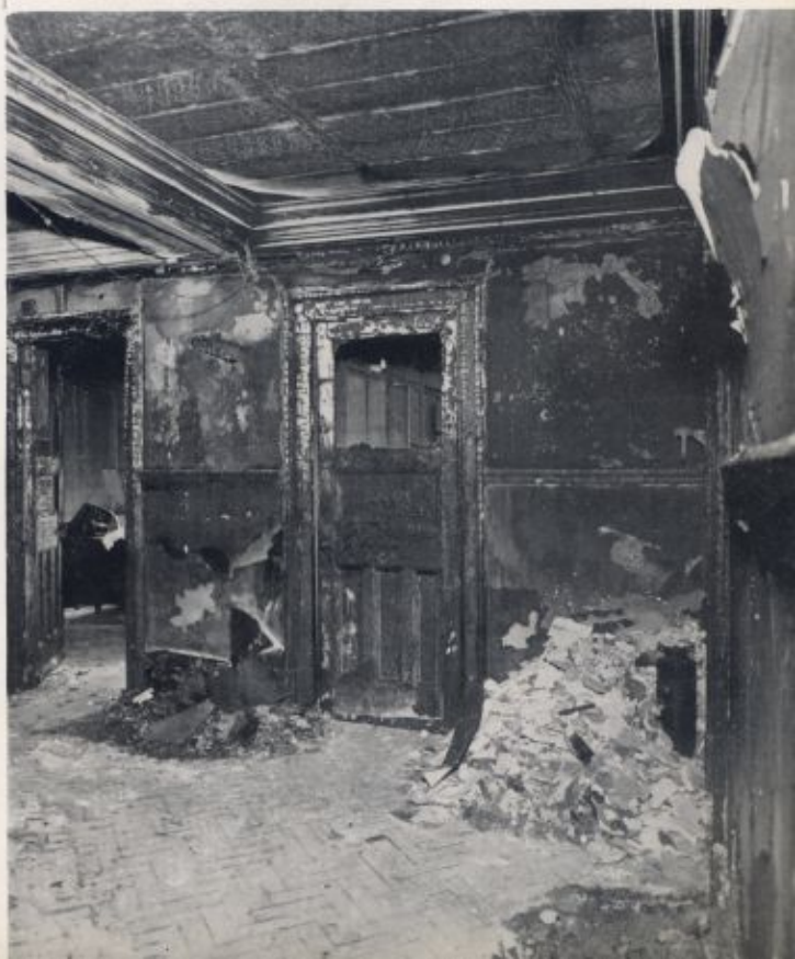
Just inside the 6th floor entrance.
